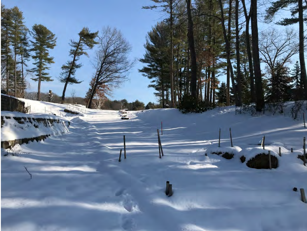
Fig 5: Slope above the manhole at Gundalow Landing/east side of the bay. Viewing east. (12-22-20)
