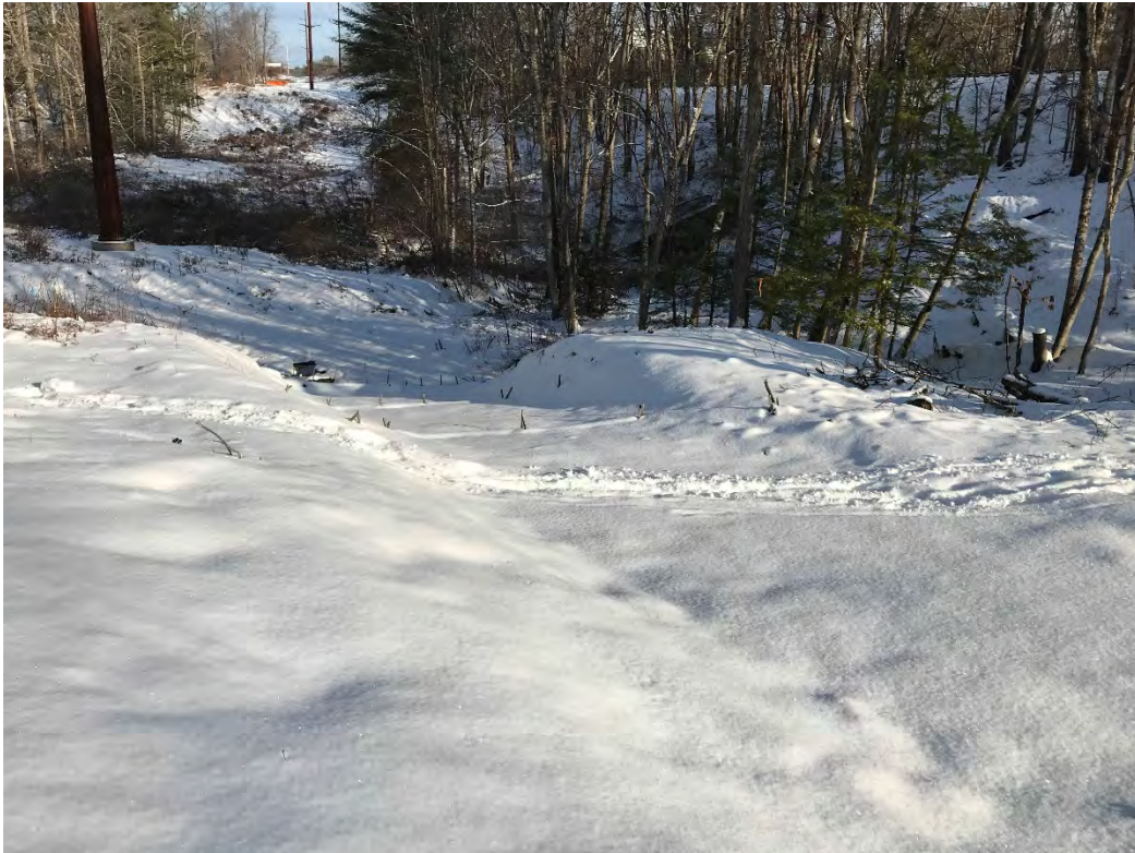
Fig 10: Lower portion of slope between Strs. 28 and 29. Viewing northeast. (12-15-20)
