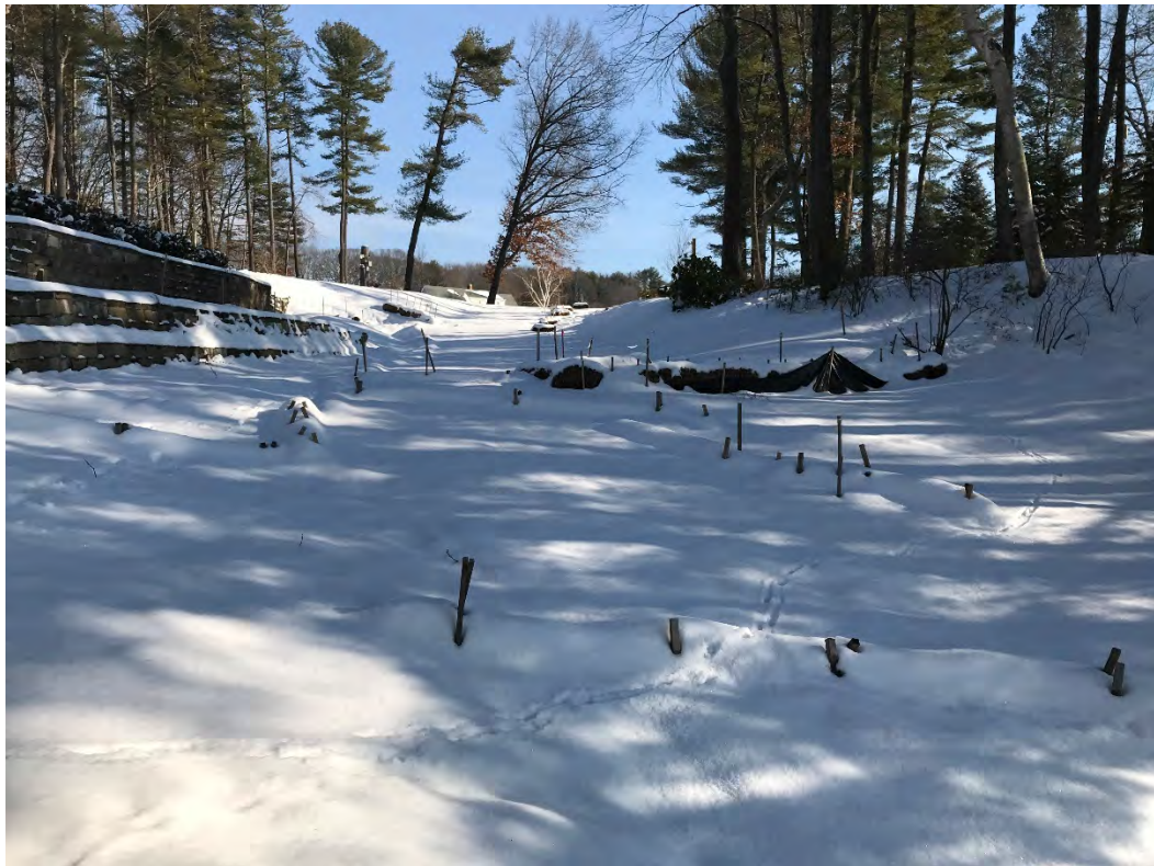
Fig 6: Slope below the manhole at Gundalow Landing/east side of the bay. Viewing east. (12-22-20)
